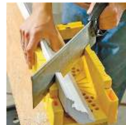
Cut cornice with saw at a 45 degree angle.
