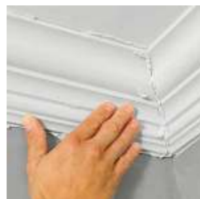
Join both cornices together, so that their profiles match. Use special adhesive to attach the items.
