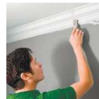
Apply filling knife to process the joints of cornices.
