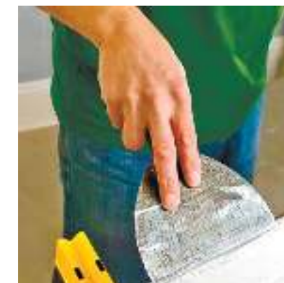
Apply adhesive along the edges at the back of the cornice as well as the mating surface.
